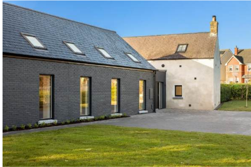
Stables Conversion to House & Extension at Seachnall Abbey, Dunshaughlin (a Protected Structure)
