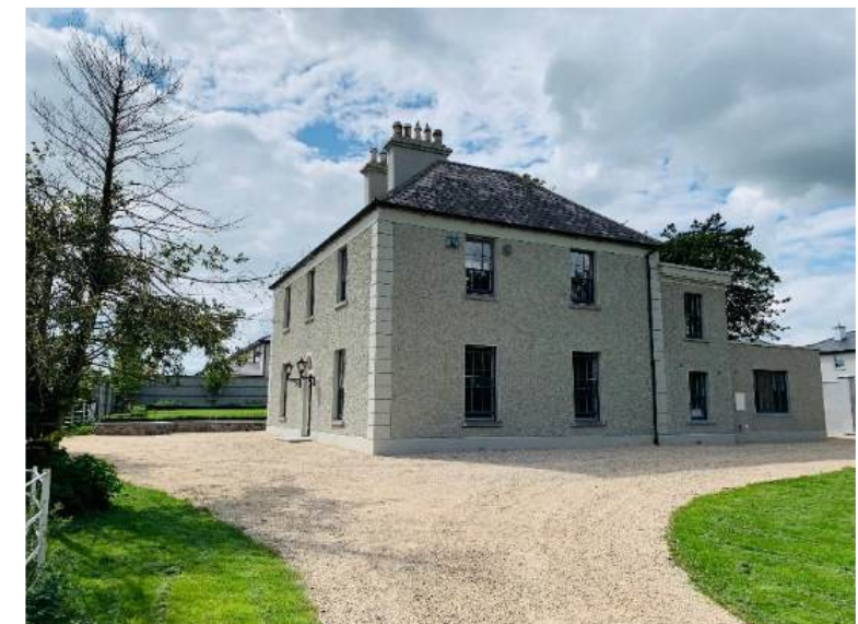
Seachnall House, Dunshaughlin (a Protected Structure)
